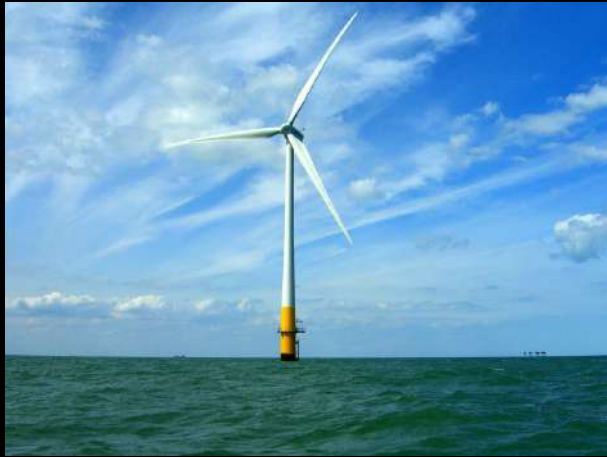
Single wind turbine
